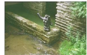
Figure 20 - Pool with Bear run in the background
