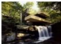
Figure 17 - Falling water, by F L Wright
