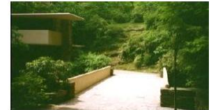
Figure 18- Falling water, Driveway over bridge to entrance
